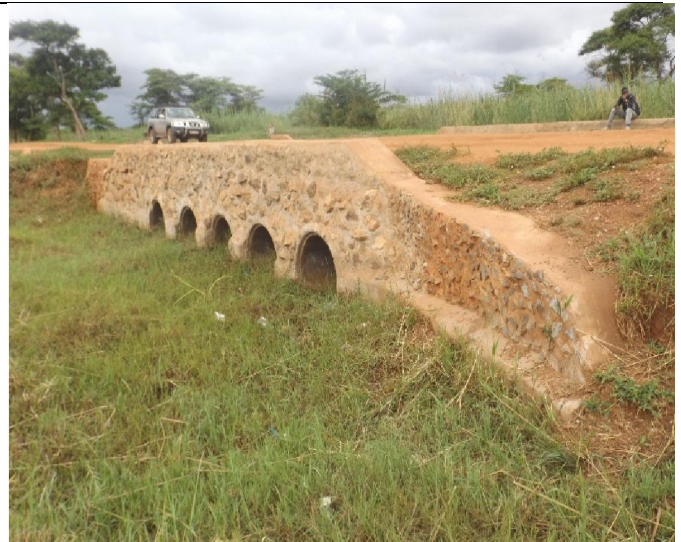
Section of the road at Kamakuti Road (D421) after the installation of the culverts-After.
