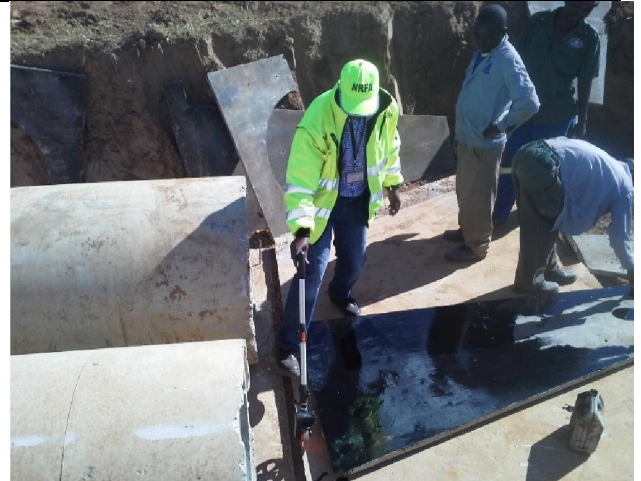
Measuring the length of the culvert
