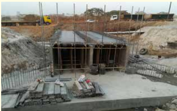
Box culvert being installed on Chingola-Kasumbalesa in Chingola-Copperbelt Province
