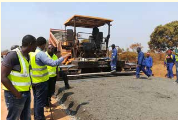
Laying of Crushed Stone Base course Chingola -Solwezi Lot 3-North-Western Province
