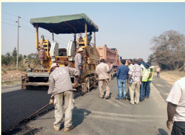
Remedial Asphalt works in rutted sections on South bound Traffic lane-Ndola-Kitwe-Copperbelt Province
