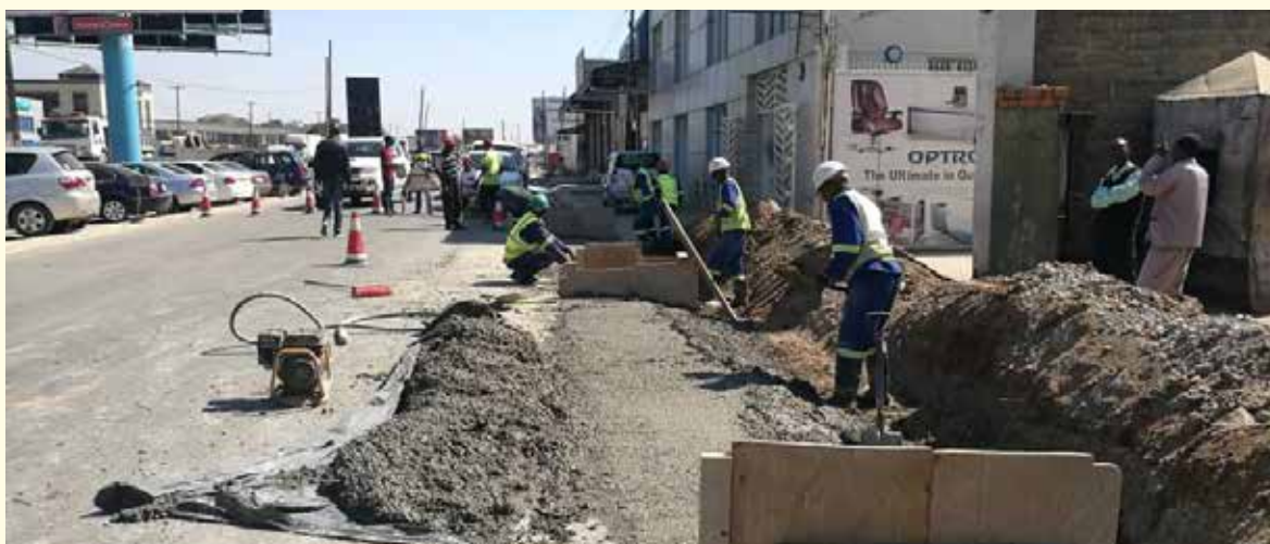
Construction of access culverts on Lumumba Road
