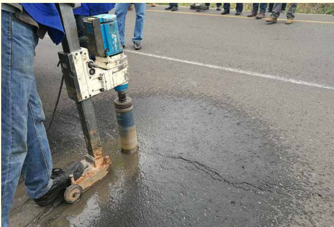
Core Drilling
