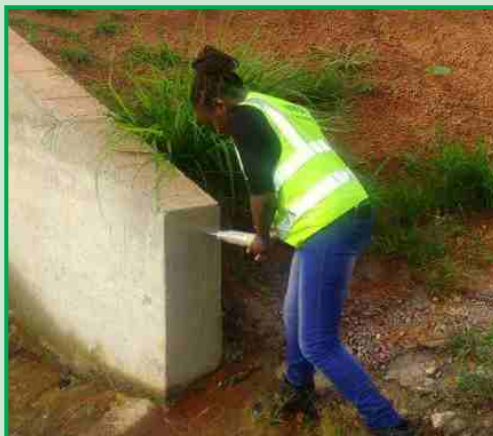
Eng. Winfridah Phiri conducting road inspections
