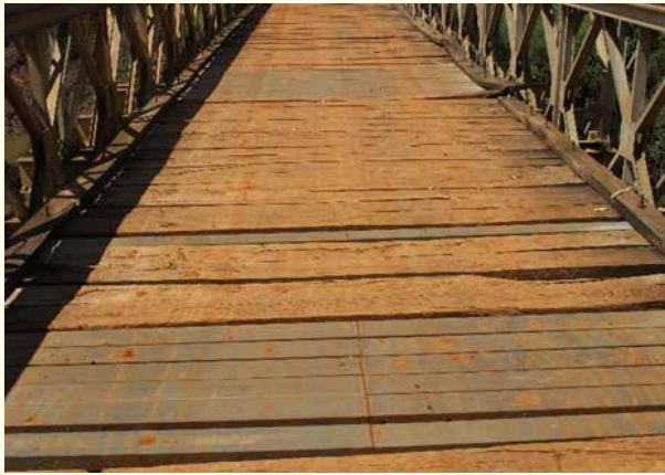
Inspection of works on the Bailey bridge
