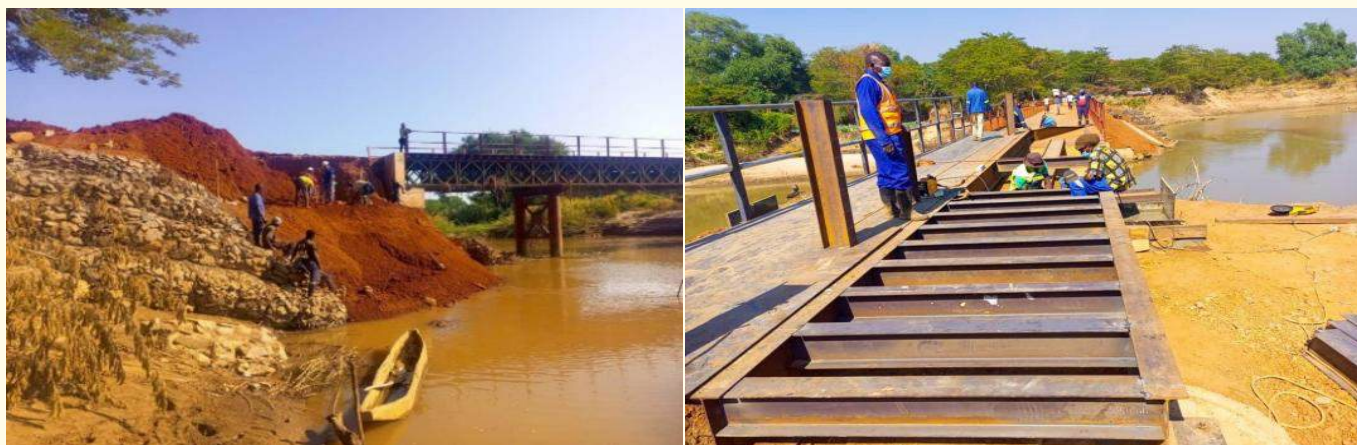
Field inspections: Luangwa Bailey Bridge Eastern Province
