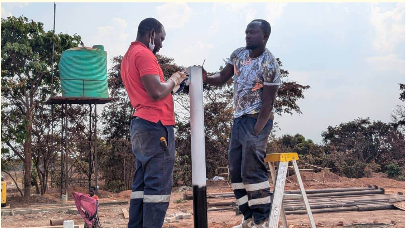
ICT personnel installing systems at the new site at Kateshi
